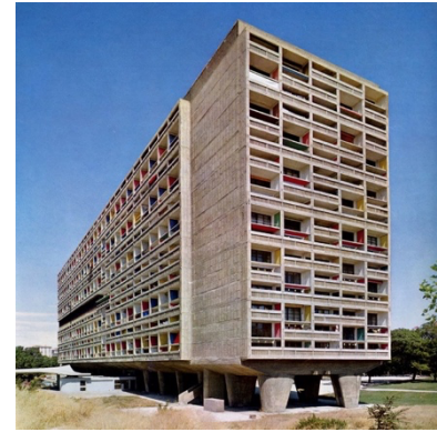
Figure 2 Unité d'Habitation with passive sunshade
