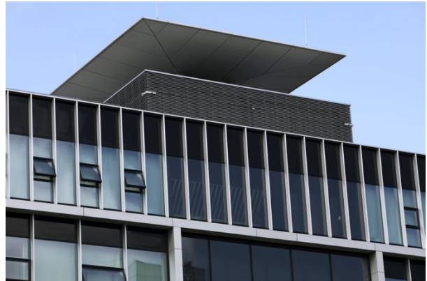
Figure 2 Ventec roof on top of the Langeveld Building
