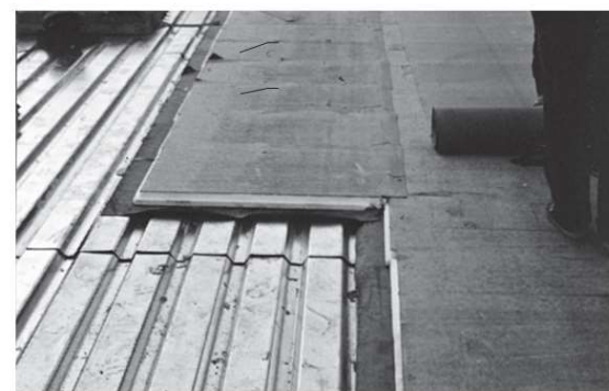
Figure 3.28 Steel roof with polystyrene foam insulation sheets with a laminated layer on either side. The roof covering is attached to the upper layer, while the lower layer functions as a vapour-retardant layer.
