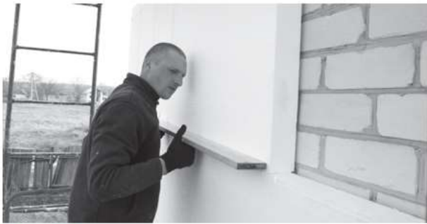
Figure 3.3 Outside insulation of a facade
