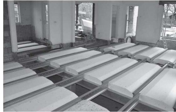
Figure 3.12 Floor insulation with EPS elements
