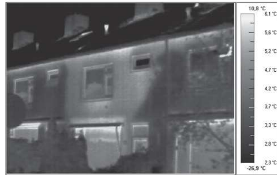
Figure 1.3 Temperature portrayed by an infrared camera
