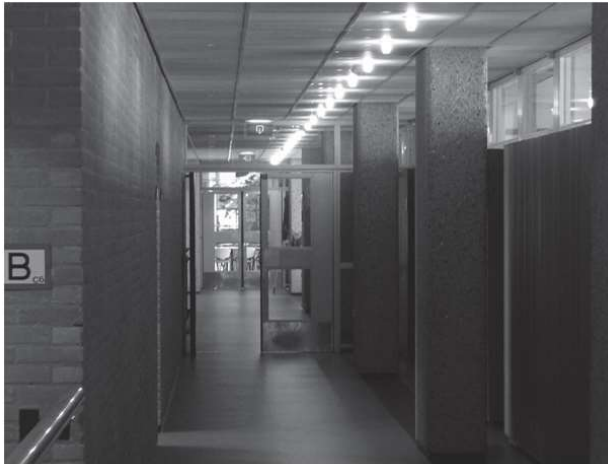
Figure 4.13 Too great differences in brightness caused by unprotected fluorescent lamps
