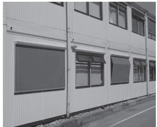
Figure 7.10 The ventilation through open windows or ventilation grids can be seriously hindered by external sunscreens
