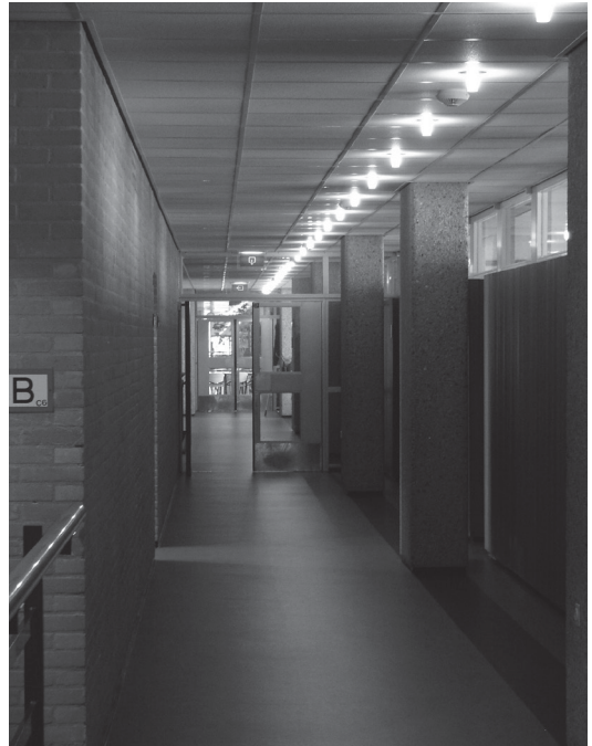
Figure 4.13 Too great differences in brightness caused by unprotected fluorescent lamps
