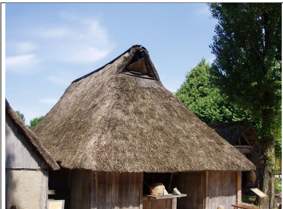
Figure 3.1.2: Example of a house of the early Middle Ages. The air exhaust can be controlled. The main original function of high openings was smoke removal, which has, without a chimney, a low effectiveness. When chimneys were being used air indoor quality and fire safety improved. (Archeon)
