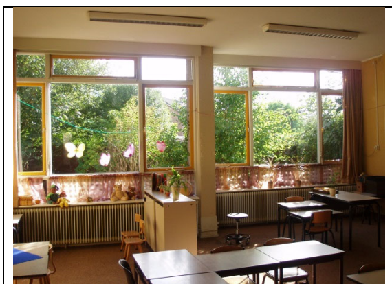
Figure 3.1.4: Example of a naturally ventilated school in Middelburg from around 1960. There are sufficient windows with different size and location and thermal mass that can be cooled down. Outside sunshade is available. The climate system was unchanged in 2006 when this picture was taken.
