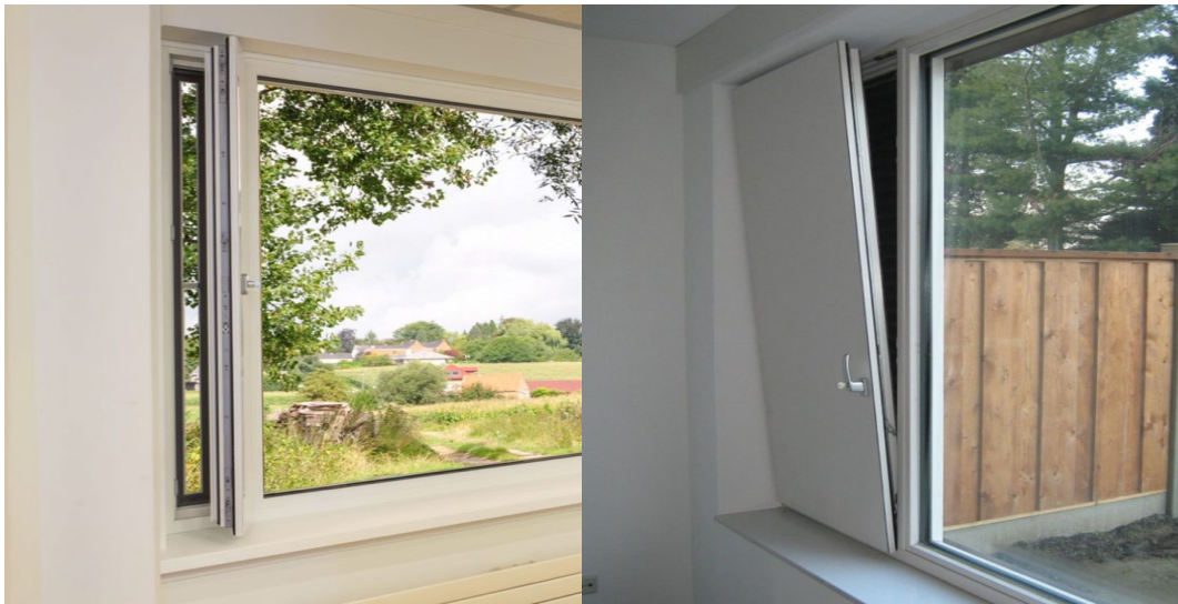
Figure 11.9: Examples of burglar-proof ventilation windows and shutters.
