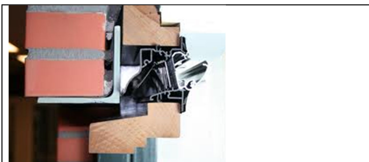
Figure 4.1.3: Example of an air inlet hidden from outside, one of the most common ways of integration of grilles in new houses in the Netherlands.
