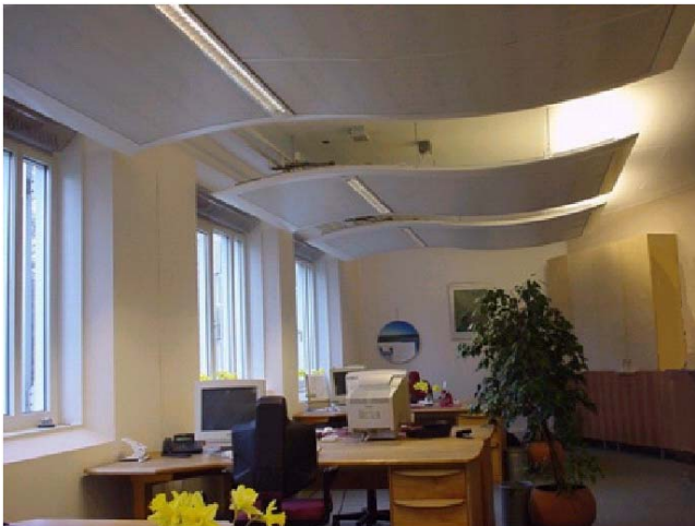
Figure 4: Air supply above a climate ceiling in order to prevent draught.
