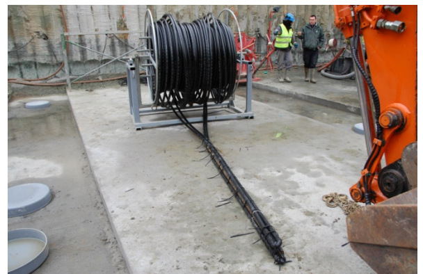
Figure 10: Borehole Thermal Energy Storage by using probes of approximately 150 meters deep.
