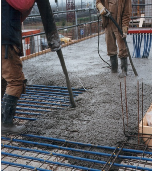
Figure 2: Traditional casting of concrete on concrete core activation piping.
